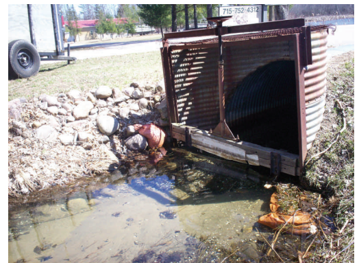
The dam by the culvert that runs under Rustic Drive has been open all winter. It regulates the water flow out of Pine Lake.
